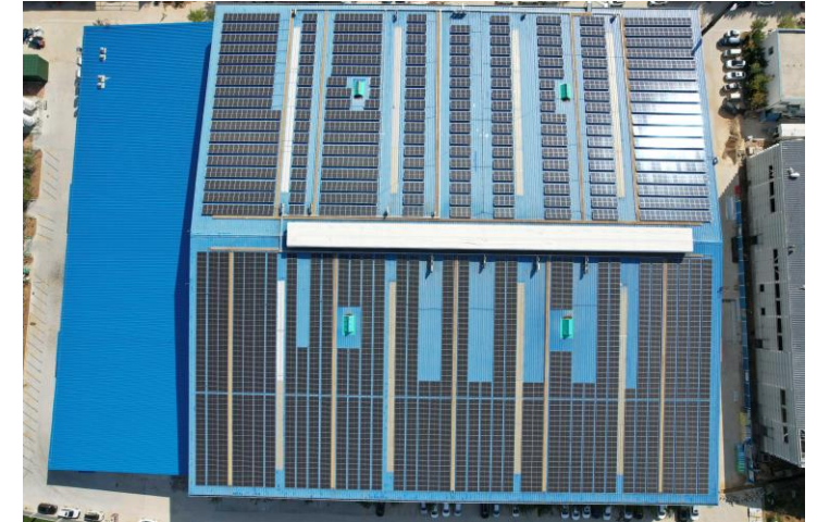
Solar panels installed at HOYA Optical Technology (Weihai) Co., Ltd. (annual generating capacity: 1,300 MWh; reduction in annual CO2 emissions: about 800 t-CO2)
