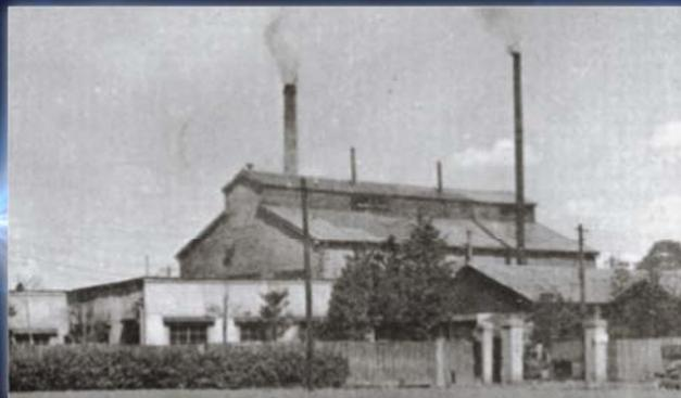
HOYA Plant at the Time of Foundation (roofs for heat exhaust and chimneys, characteristics of glass manufacturing plant, are visible)
