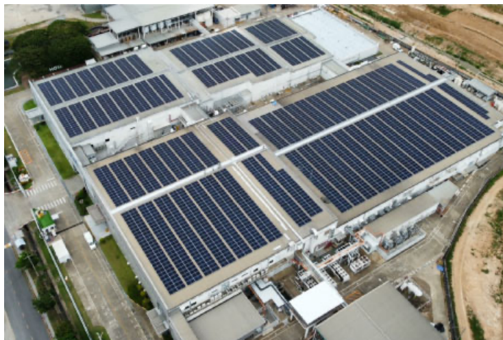
Solar panels installed at HOYA LAMPHUN LTD. (Annual generating capacity: about 2,200 MWh; Annual CO 2 reduction volume: about 1,000 t-CO 2 )
