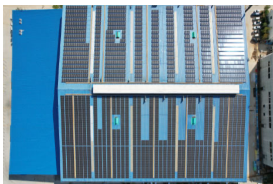
Solar panels installed at HOYA Optical Technology (Weihai) Co., Ltd. (annual generating capacity: 1,300 MWh; reduction in annual CO 2 emissions: about 800 t-CO 2 )
