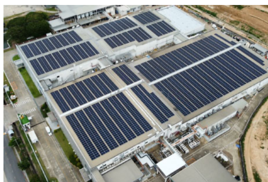
Solar panels installed at HOYA LAMPUN LTD. (Annual generating capacity: about 2,200 MWh; Annual CO 2 reduction volume: about 1,000 t-CO 2 )
